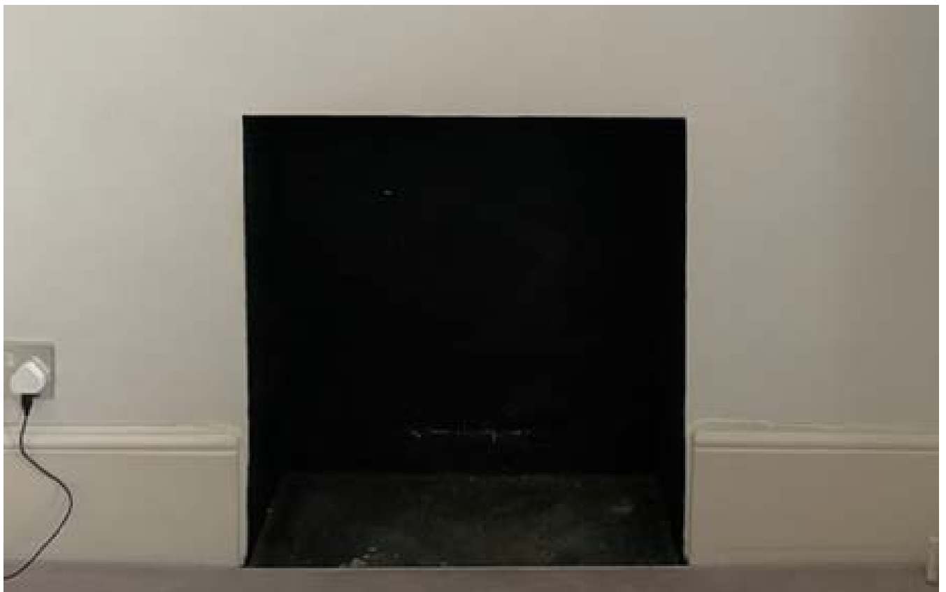
Figure 8 Chimney breast to be boarded over in master bedroom. Skirtings to match.
