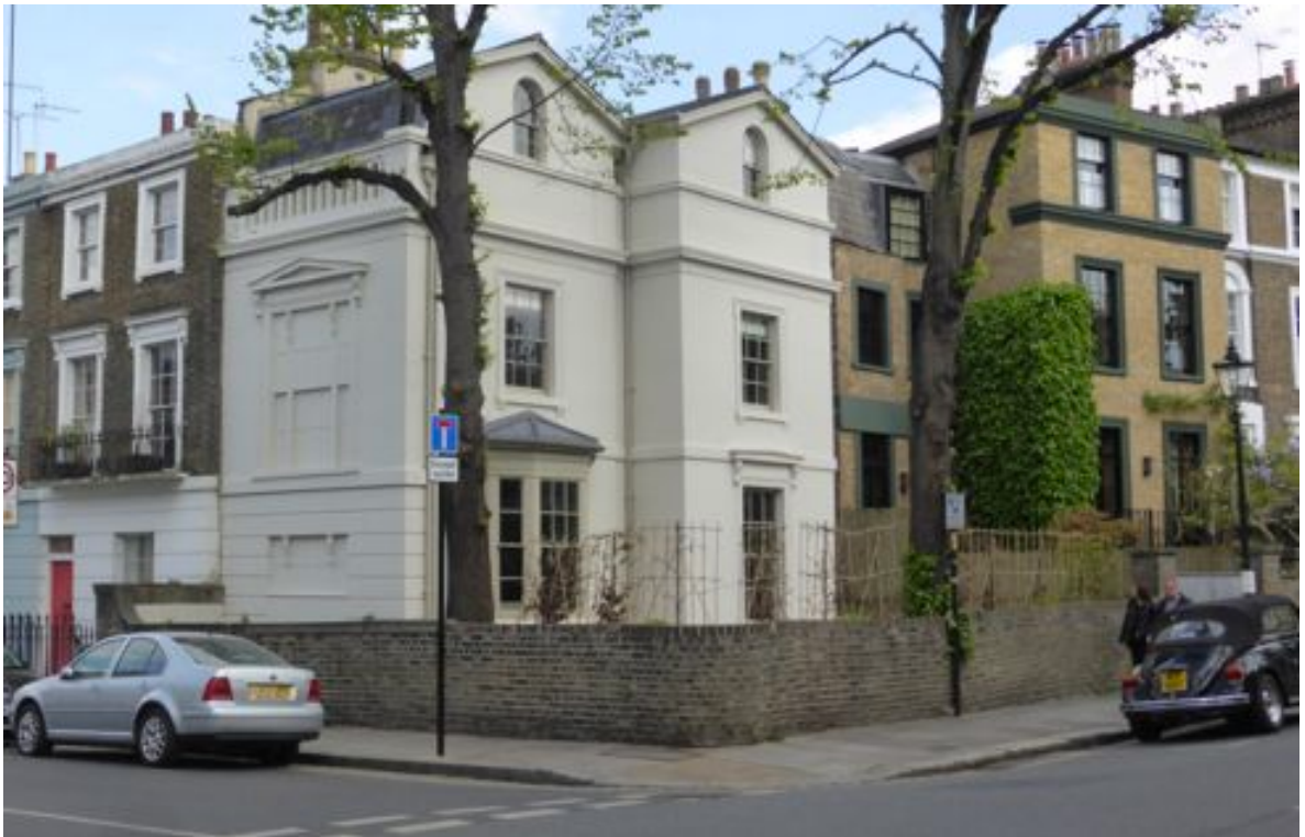
Fig. 9 North and West boundary wall
