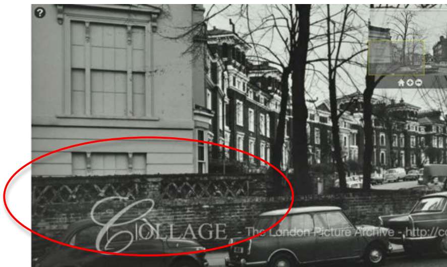
Fig.3 Number 23 Gloucester Crescent detail of North wall circa 1967.
