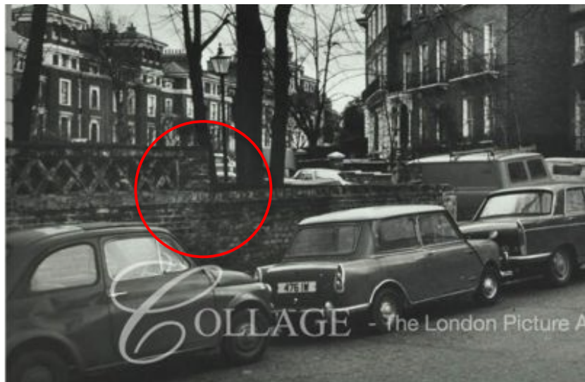
Fig.7 Detail of the truncated end of the original wall circa 1967.
