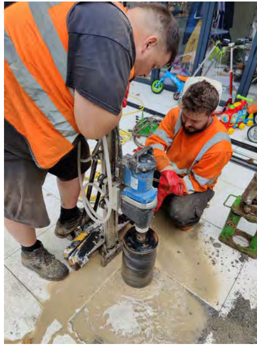
BH01 Concrete Coring 13/10/21
