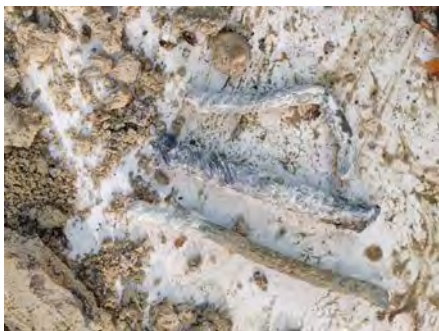
BH01 rebar from base of concrete 01/11/21
