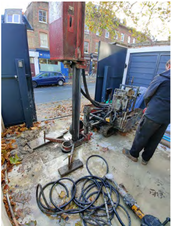
BH01 conventional drilling with Trent tracked rig.01/11/21
