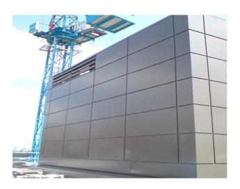
Acoustic Panels have a plain exterior surface and a perforated inner surface with an acoustically absorbent media being contained between the two skins. The inner perforated surface allows exposure of the acoustically absorbent media to the noise source in order to reduce reverberation within the area around the enclosed machinery. If necessary, the external surface of the panel can be acoustically damped to eliminate local resonances.
