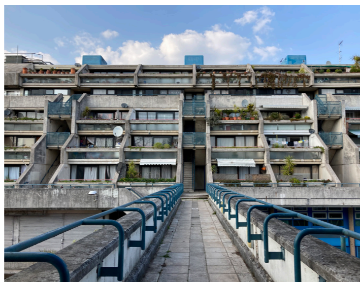
Fig. 7.5: Alexandra Road Estate.
