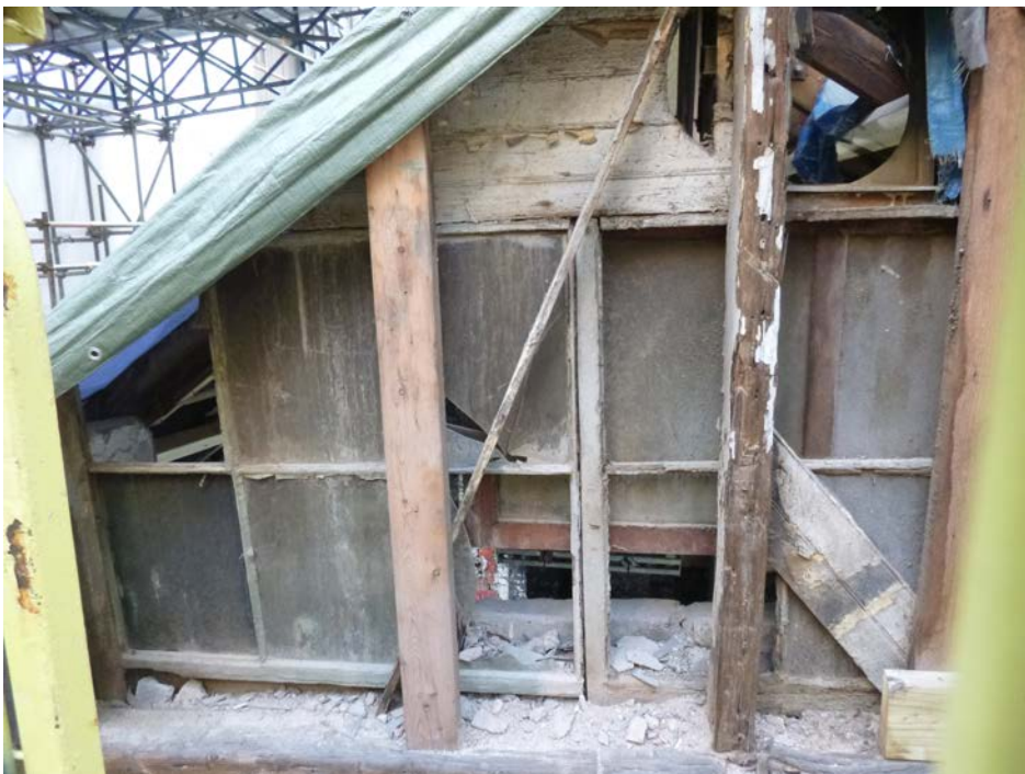
East gable, 2017. The poorly fitted window appears to be re-used from elsewhere
