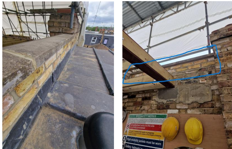
Party wall between 55 (Application Property) and 57 Princess Road. Raised wall highlighted.
