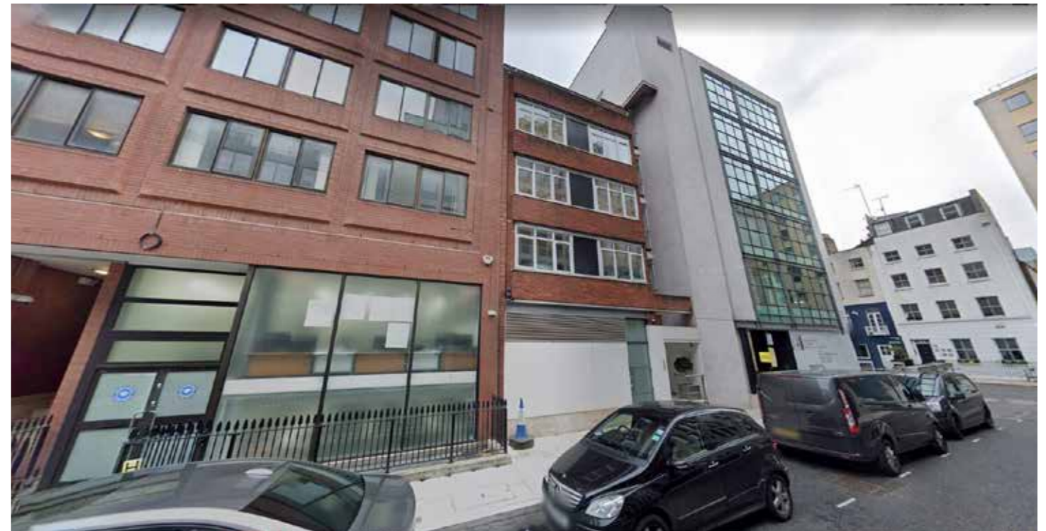
CHITTY STREET - Rear entrance showing area for new window
