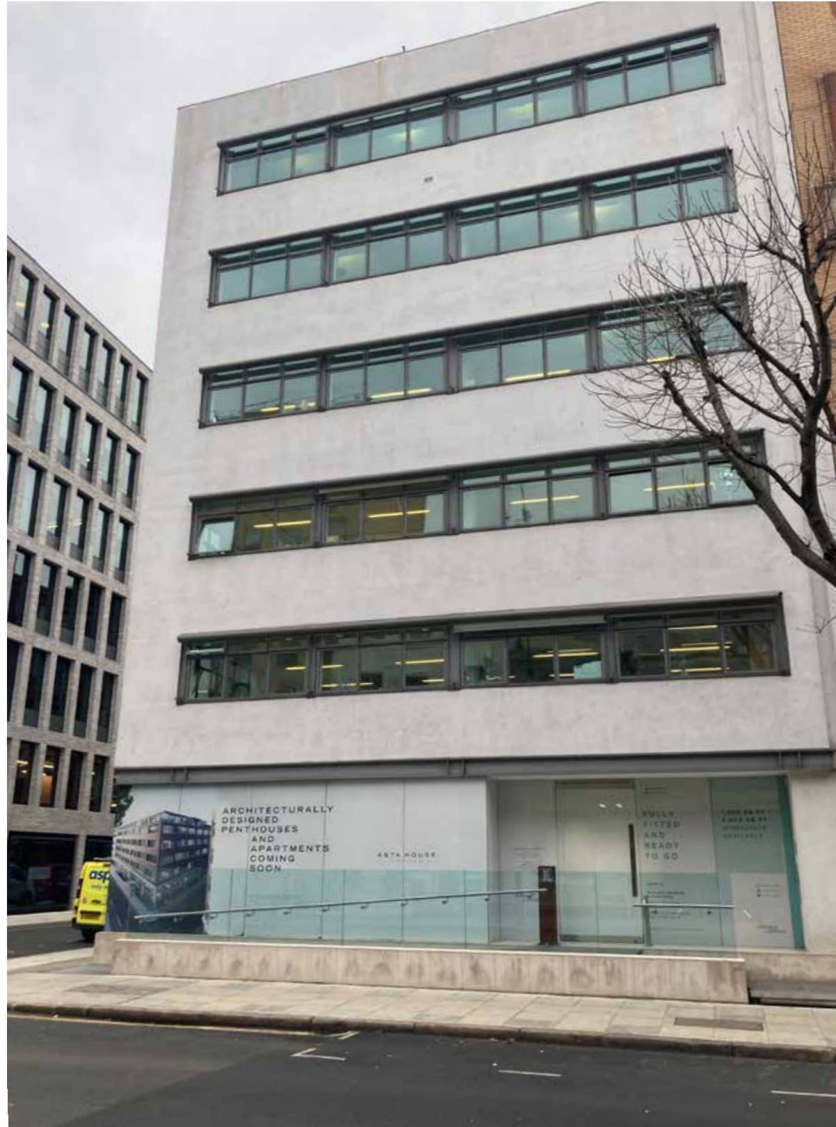
CHARLOTTE STREET - Front entrance
