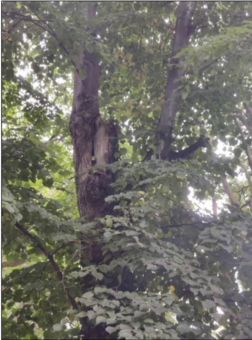
Photograph 3: Decay at pollarding point of T7
