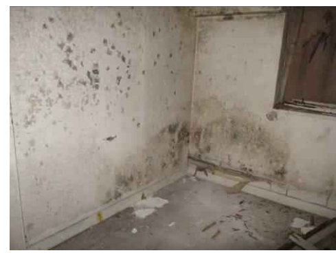
Mould growth and rising damp to staff accommodation
