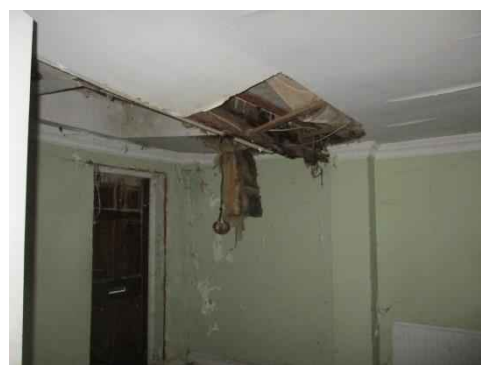
Collapsed ceiling
