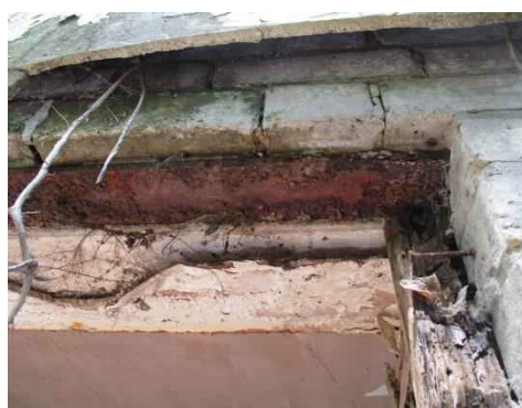
Corroded window lintol
