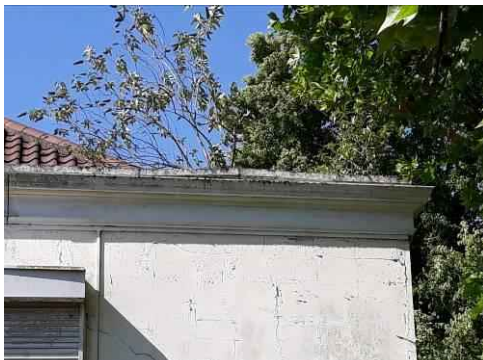
Vegetation growth to the north-east corner parapet of the main building
