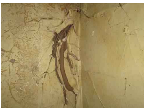
A root has penetrated the building fabric
