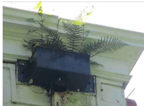
Vegetation growth within a cast iron hopper
