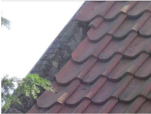
Missing pantiles to staff accommodation roof
