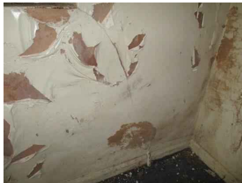
Penetrating damp in the staff accommodation
