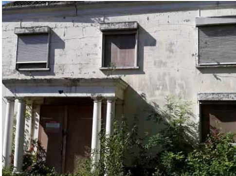
Sulphate attack on east elevation of the main building
