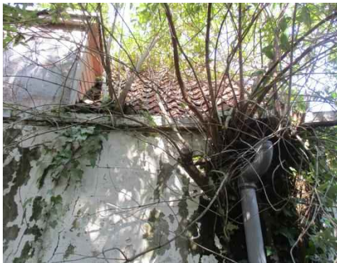
Buddleia plants causing damage to structure and rainwater goods
