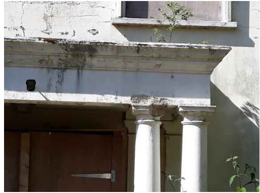
Dislodged columns and damaged cornice to porch
