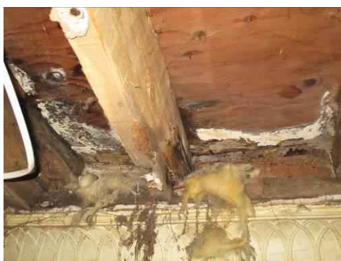
Rot to first floor timber floor joist
