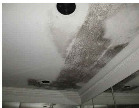
Damp penetration from roof
