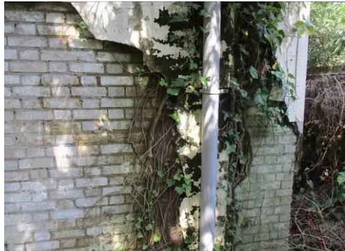
Section of de-bonded render and invasive vegetation
