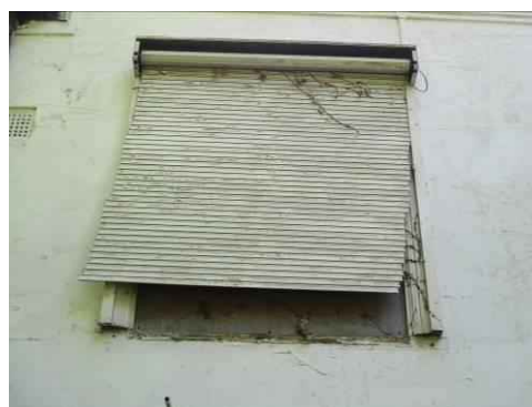
Defective roller shutter
