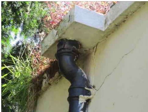
Cracked cast iron swan neck detail
