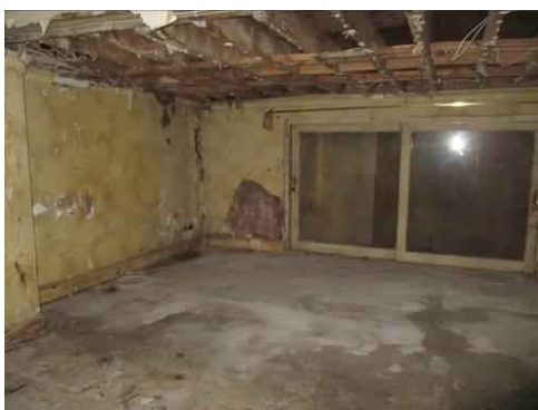
Plaster ceiling removed adjoining reception
