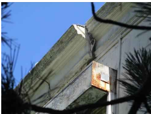
Very loose cornice section to the west parapet
