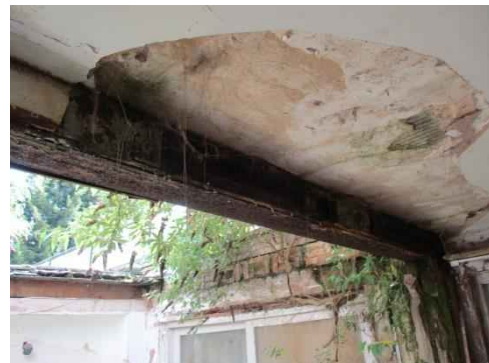
Corroded steel beam
