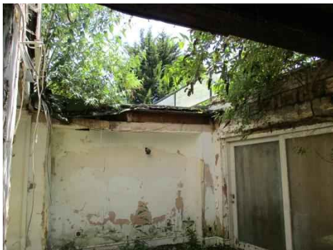
Collapsed roof / ceiling over reception area
