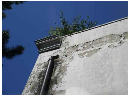
Disconnected uPVC downpipe causing severe damage to wall below
