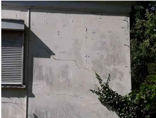
A stepped crack to the north-east corner
