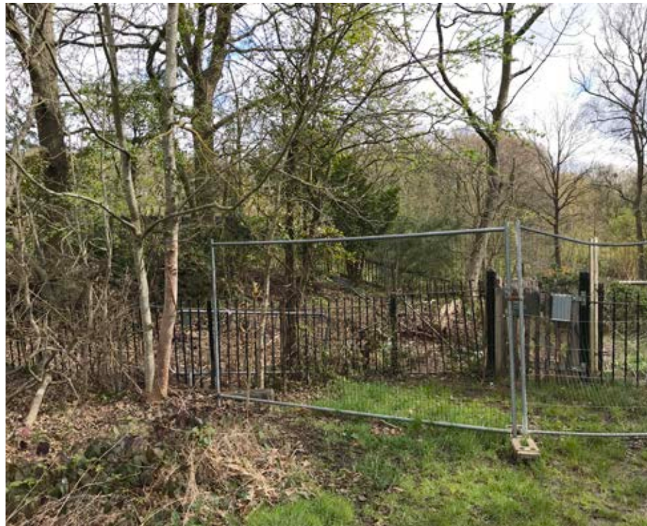
1.Existing low gate & fence at the rear
