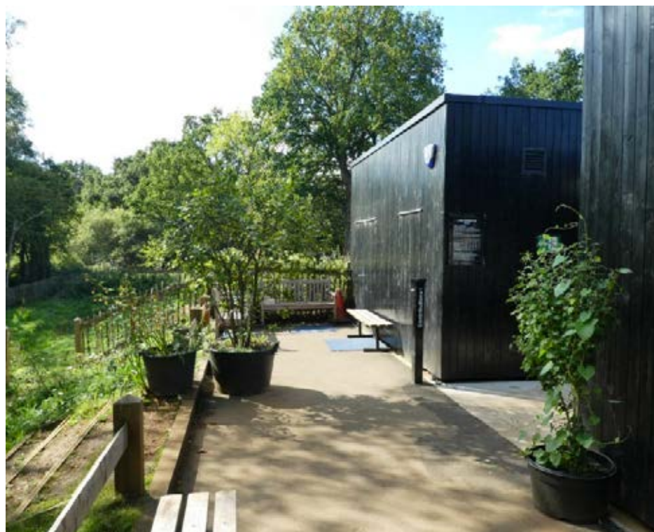
3.Existing timber clad buildings (east)
