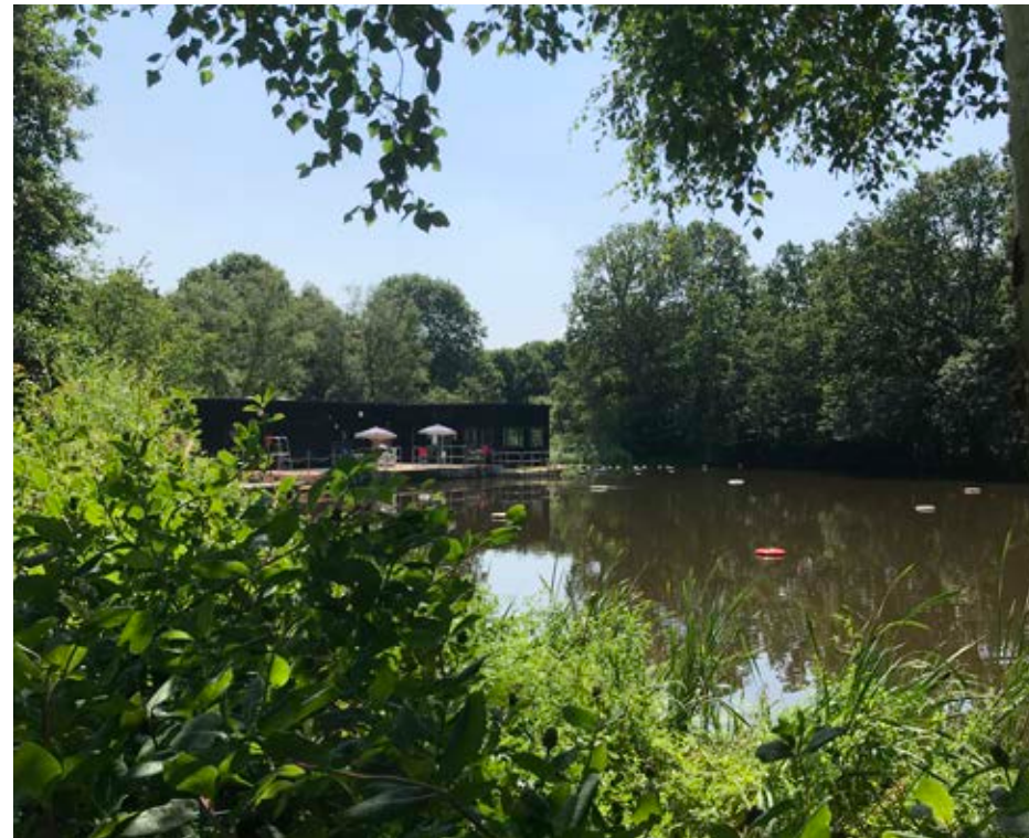
2.Existing changing & Lifeguards' buildings (west)
