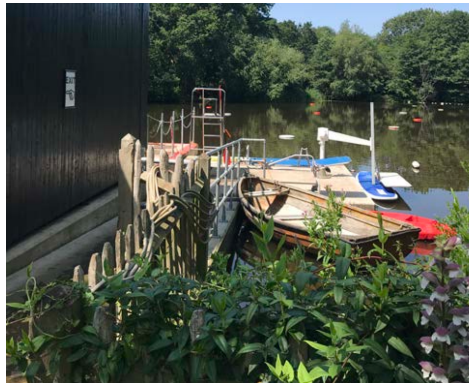
4.Existing ramped access to a concrete platform with/ a hoist for access into the water
