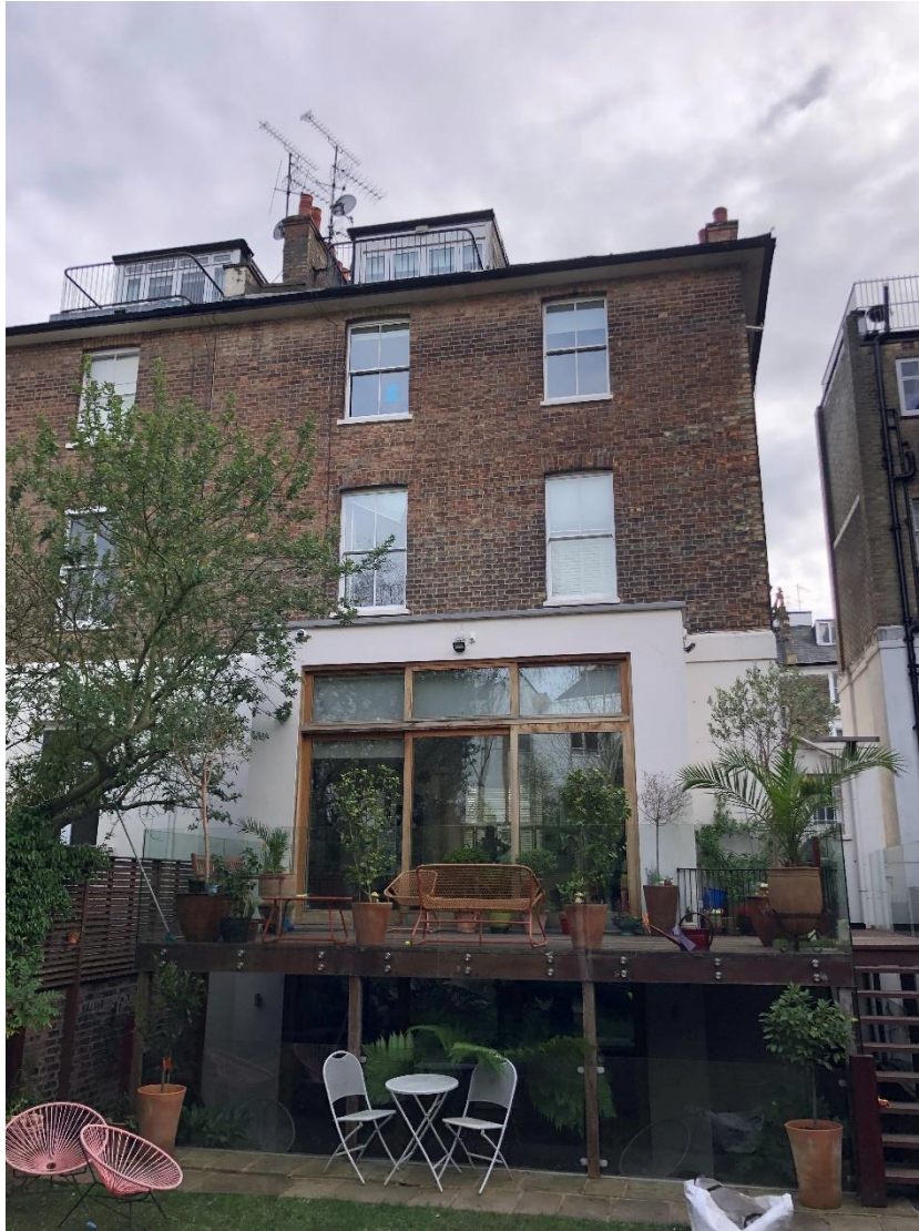
Image: 2 Thurlow Road – Rear elevation
