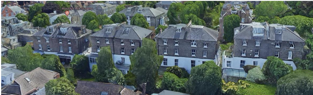
Aerial image: contextual rear elevation and roof treatment to Thurlow Road (angle 2)
