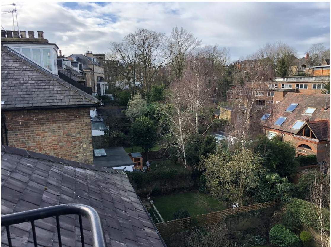
Image: a variety of later extensions and alterations can be seen to the rear of properties along the north side of Thurlow Road
