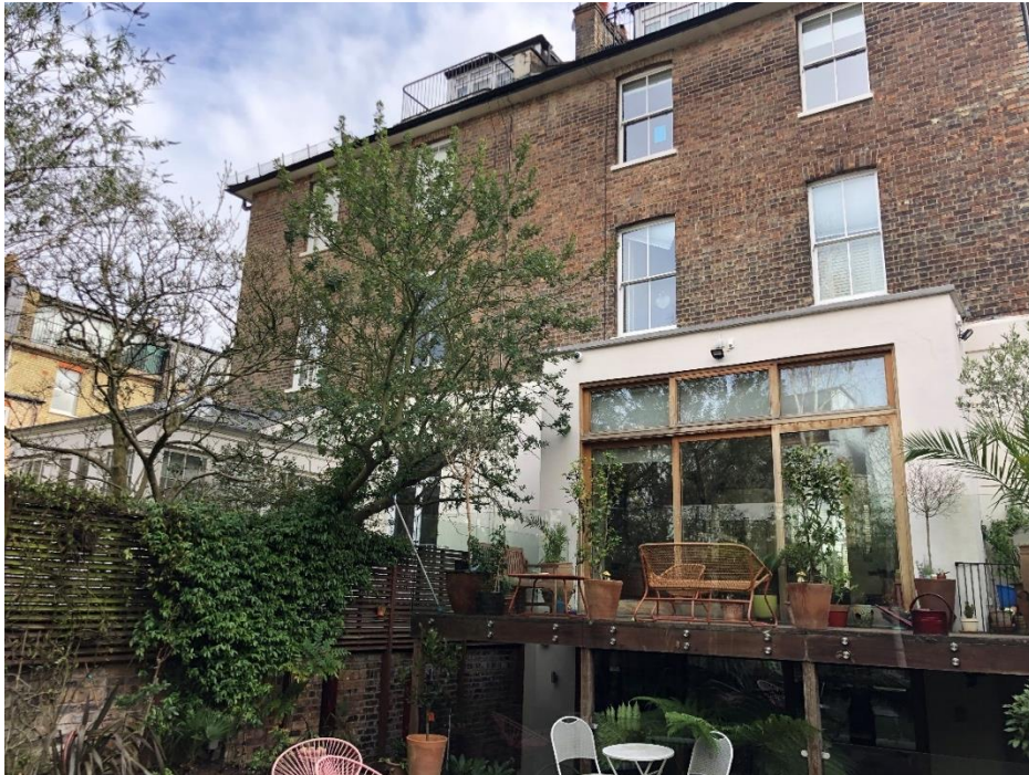
Image: 2 Thurlow Road – Rear elevation showing existing relationship to 1 Thurlow Road
