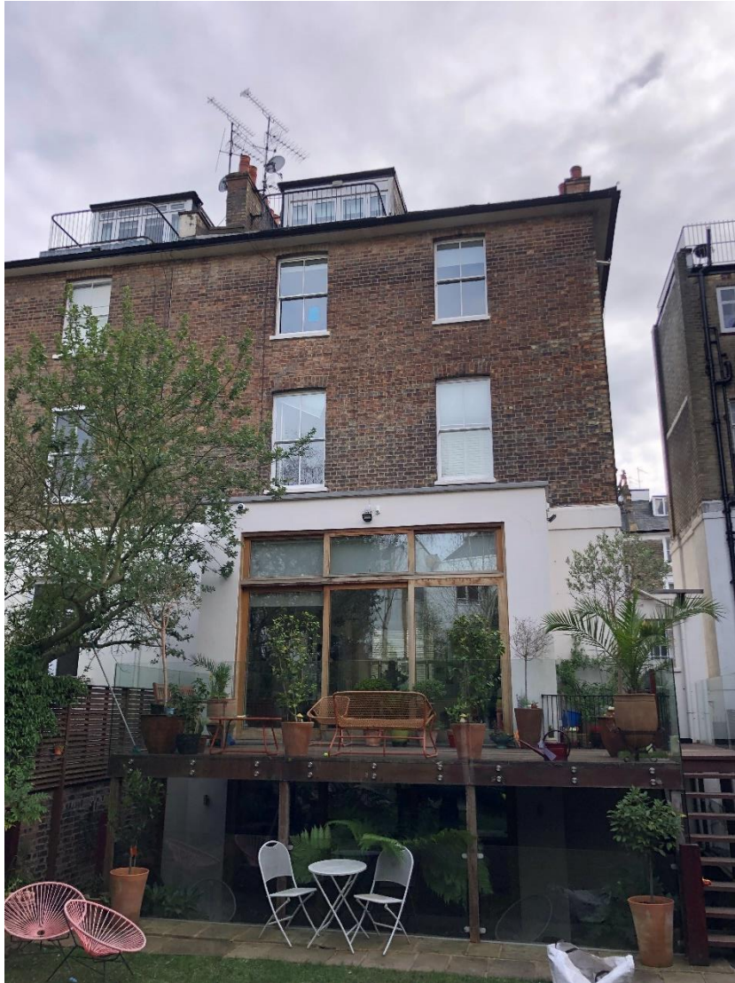
Image: 2 Thurlow Road – Rear elevation
