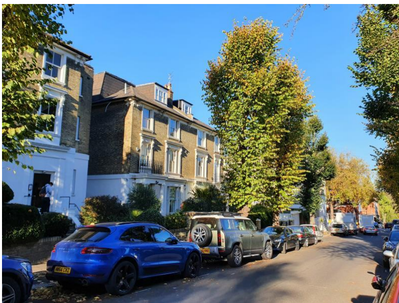
Photo 1 - view of 2 Thurlow Road seen centre with two street tree common lime (T19 & T20) in front of the property:
