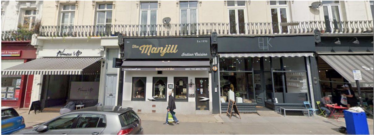
2. Photo of existing neighbouring shopfronts
