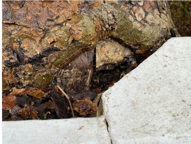
Photographic plate showing coping stones on front garden wall, damage to tree stem and embedded concrete from coping stones.
