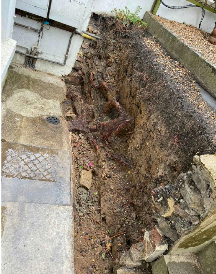
Photographic plate showing the extensive root system immediately behind and below the failed retaining wall.
