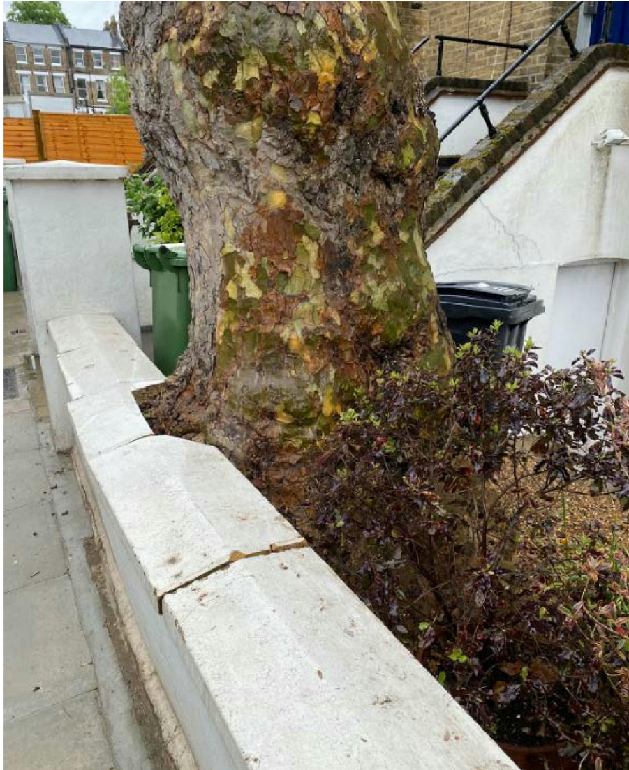
Photographic plate showing front garden wall, coping stones displaced by tree stem, and bowing in wall from pressure from tree stem.
