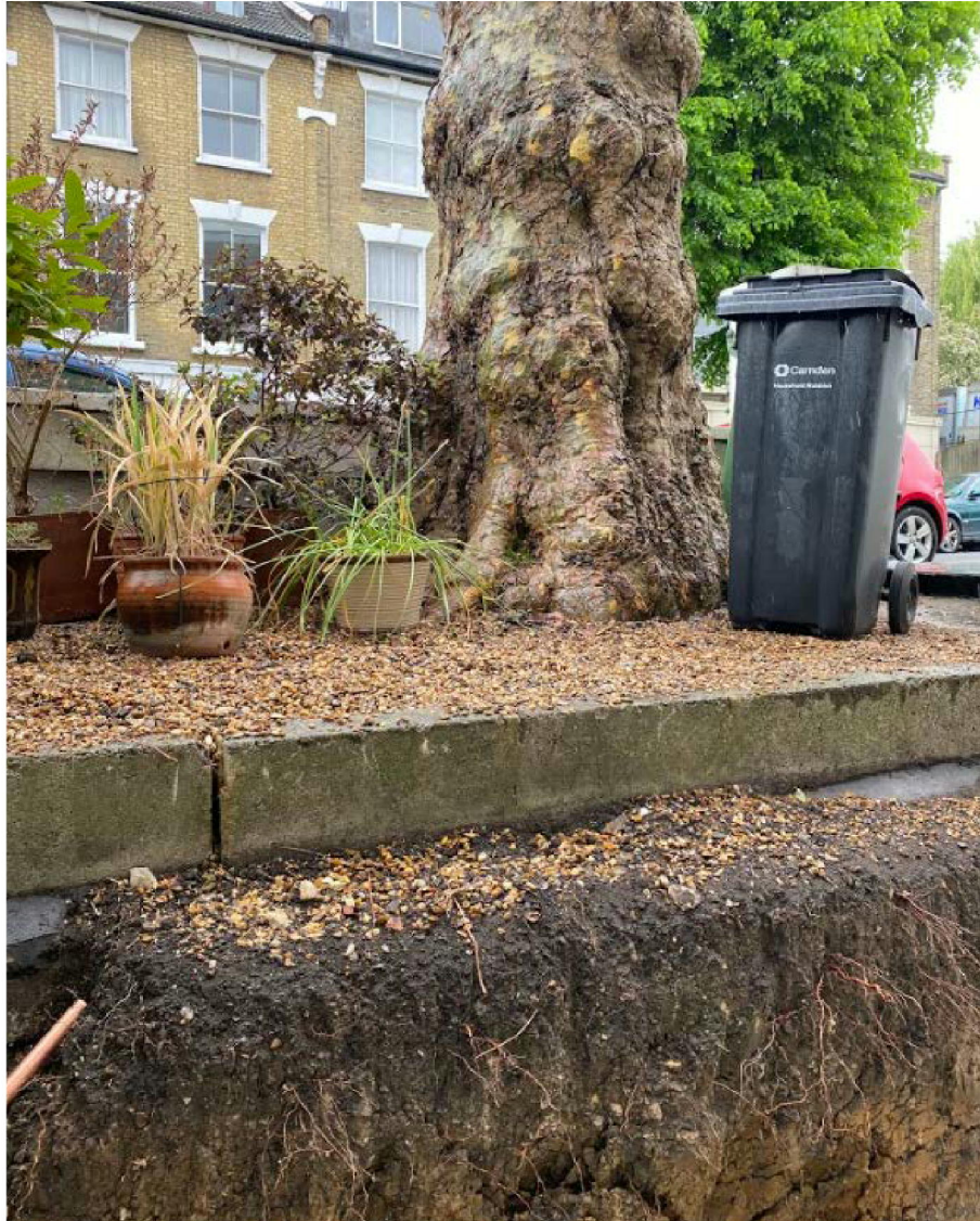
Photographic plate showing the tree's stem and proximity to the failed retaining wall
