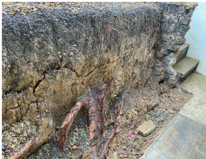
Photographic plate showing the soil bank behind the failed retaining wall.
