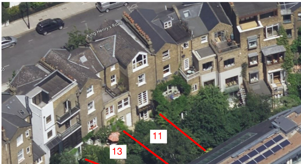
Image 1 – aerial view of host and adjoining properties (nos. 11 and 13) in wider rear terrace
