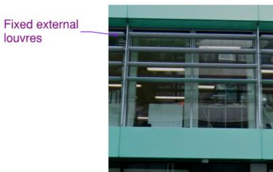
Figure 6 Fixed external louvres (brise soleil) for solar shading
