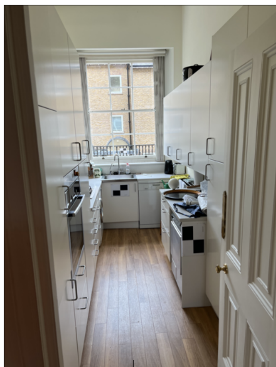
strip out existing kitchen units, appliances and floor finish
