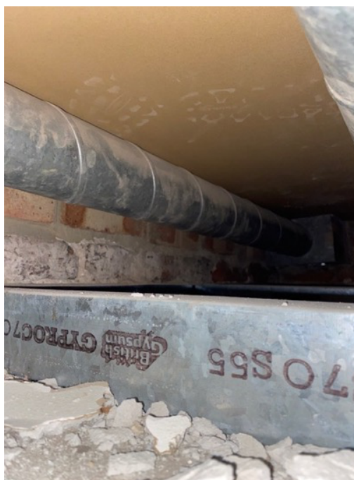
Inspection hole to top of wall showing Common Bricks and Modern Suspended Ceiling
