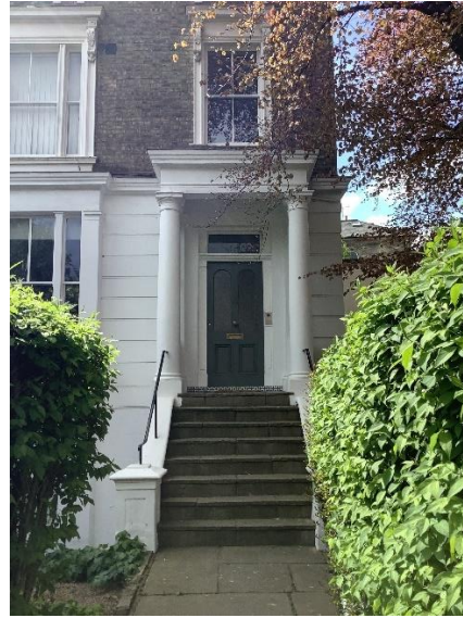
Front elevation of main property
