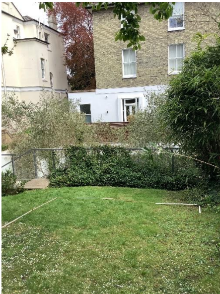
Rear elevation of main house
