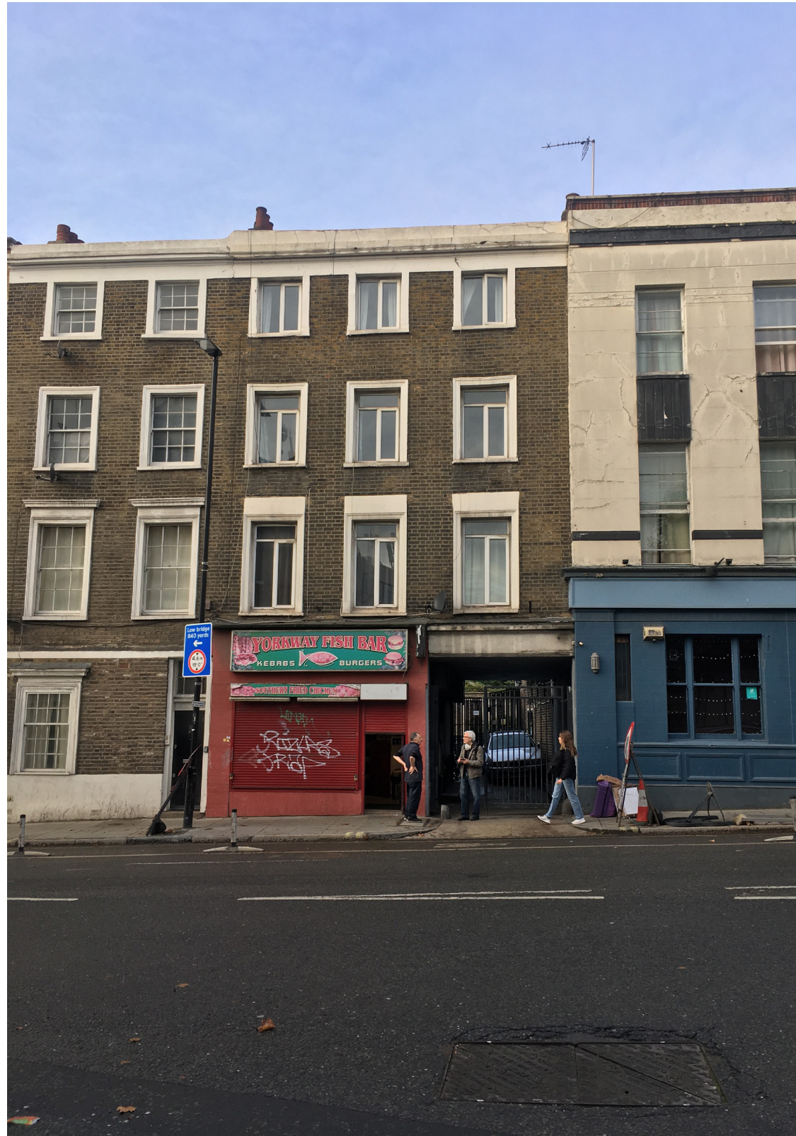
Existing front elevation of 15 York Way
