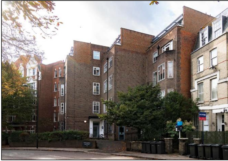
Figure 2: Existing Building and adjacent buildings (street view)
