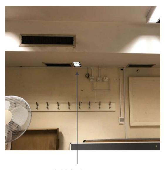
New AP fixed to modern plasterboard ductwork bulkhead on ceiling mounted bracket.
