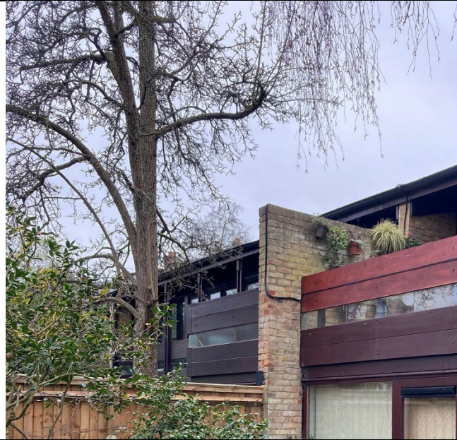
Existing privacy wall between Nos.2 and 3 The Old Orchard. This is significantly higher than the trellis at No 1.
