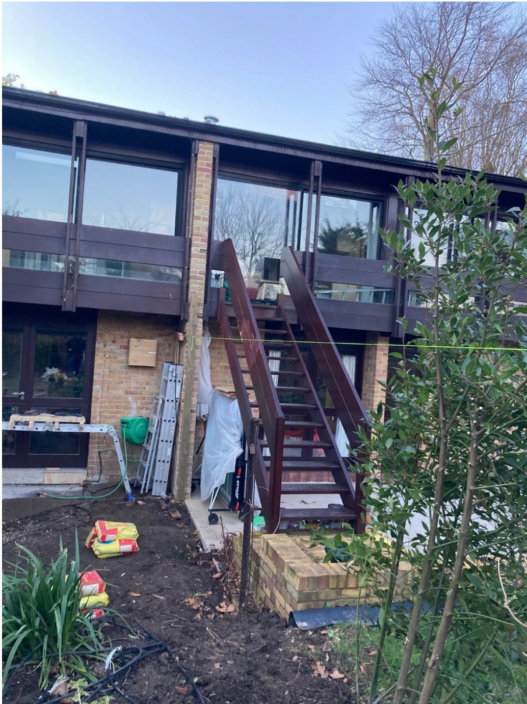
Photo of brick steps base of flight of steps
