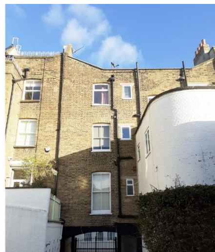
South façade facing Erskine Mews
