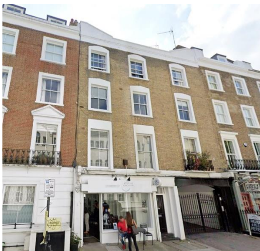
North façade facing Erskine Road
