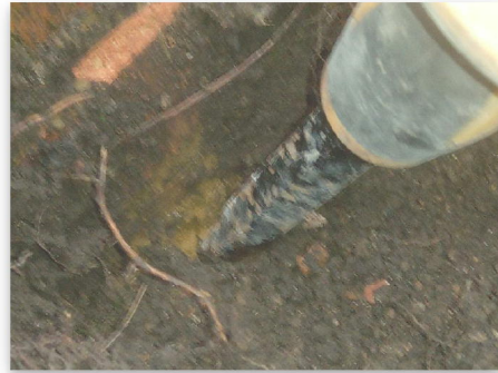
Fig 1.2: Trial Hole 1 Footing
