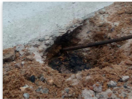
Fig 2.2: Trial Hole 2 Footing
