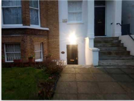
Fig 7.1: Steps which MH is located beneath
