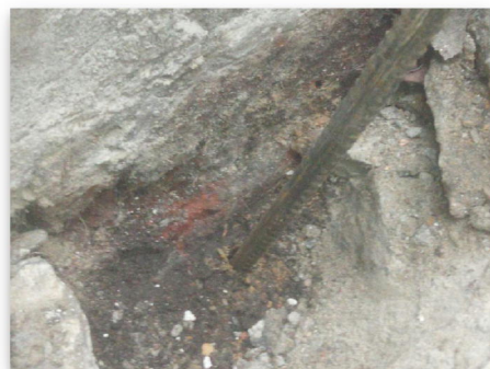
Fig 3.2: Trial Hole 3 Footing
