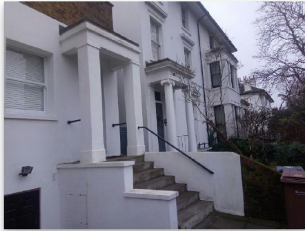
Fig 1.1: Trial Hole 1 Location
