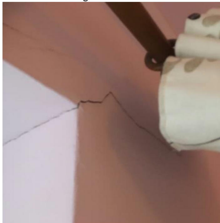
Rear Bedroom - Garden floor flat - rear wall
