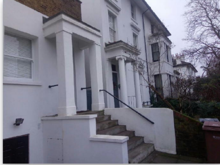
Fig 1.1: Trial Hole 1 Location
