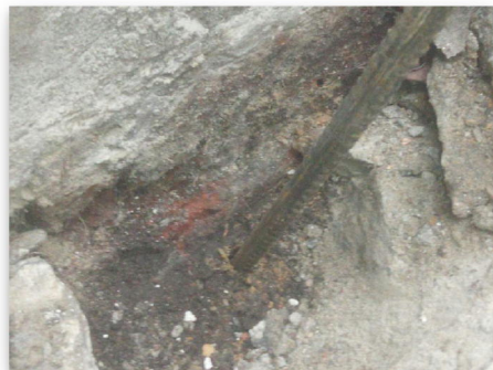
Fig 3.2: Trial Hole 3 Footing
