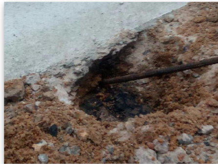
Fig 2.2: Trial Hole 2 Footing
