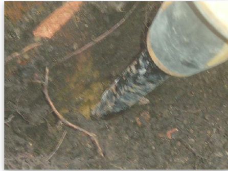
Fig 1.2: Trial Hole 1 Footing
