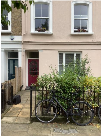
Front elevation of main property
