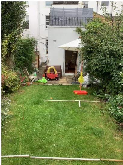
Rear elevation of main house
