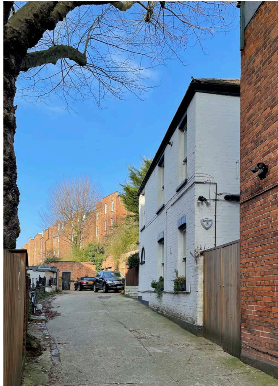
The Coach House viewed along accessway from Fawley Road
