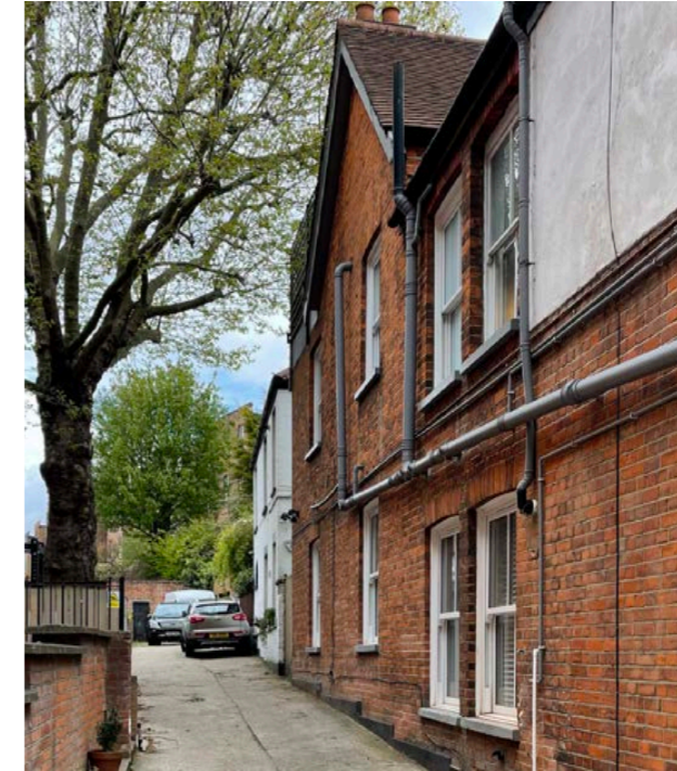
View from access yard along Ramsey House - only eaves of Coach House are visible
