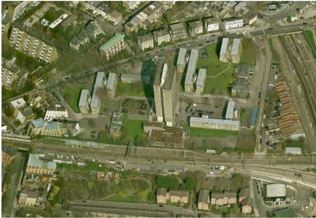
Figure 1: Oblique aerial photograph of the pre-development site looking north (Source: Microsoft Bing)
