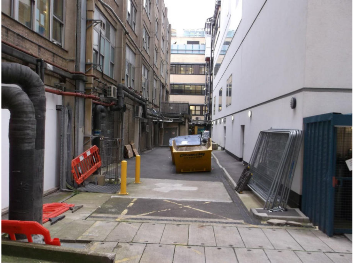
Plate 6: View of the courtyard and vehicle access to the rear of the Frontage Building, looking south-west
