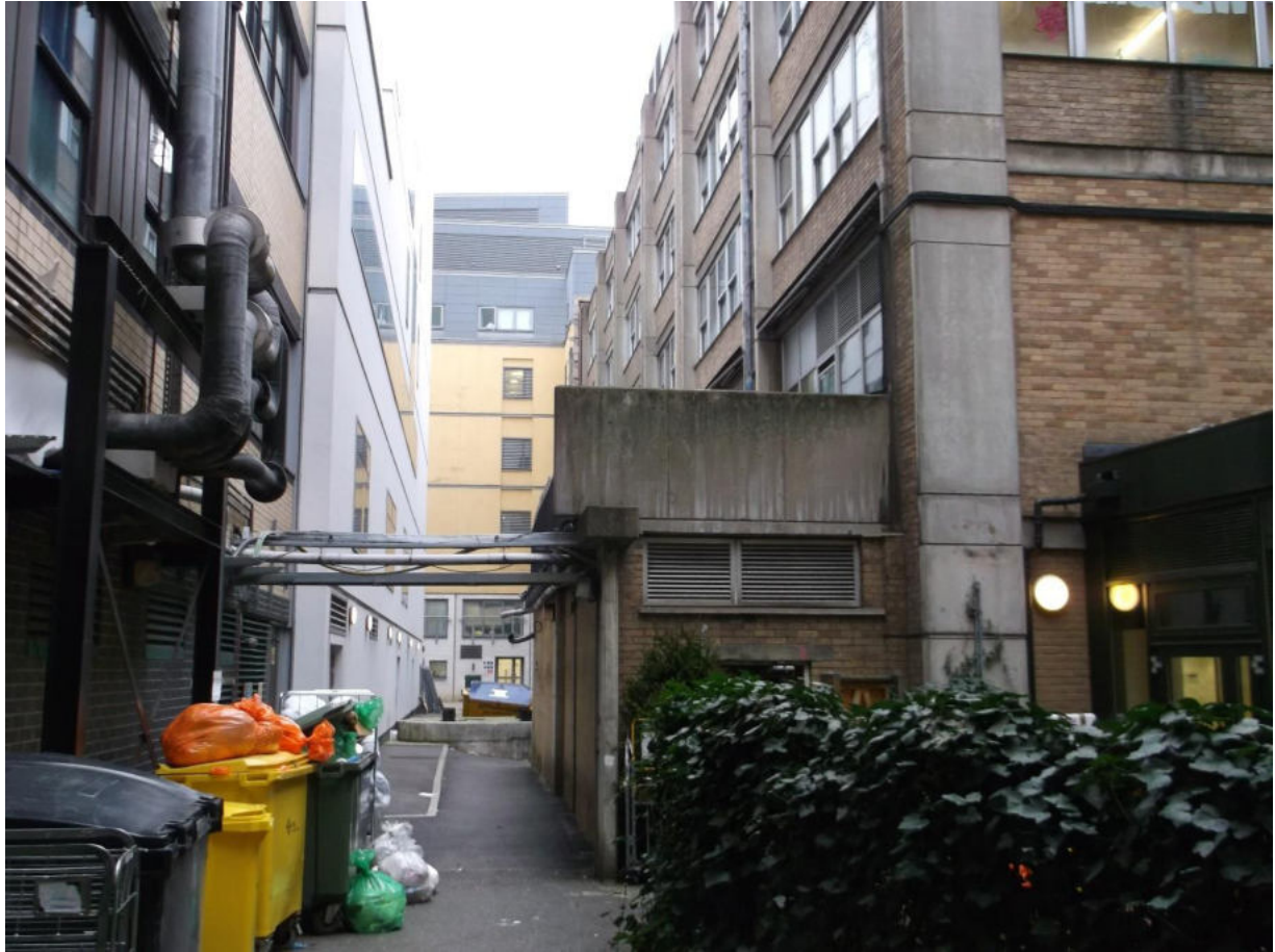
Plate 5: View of the courtyard and vehicle access to the rear of the Frontage Building, looking north-east
