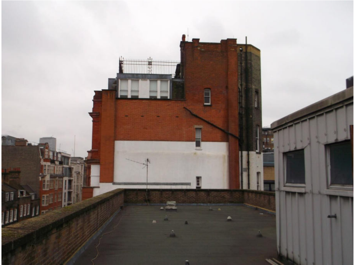
Plate 10: View of the rooftop of the Frontage Building, looking south-west
