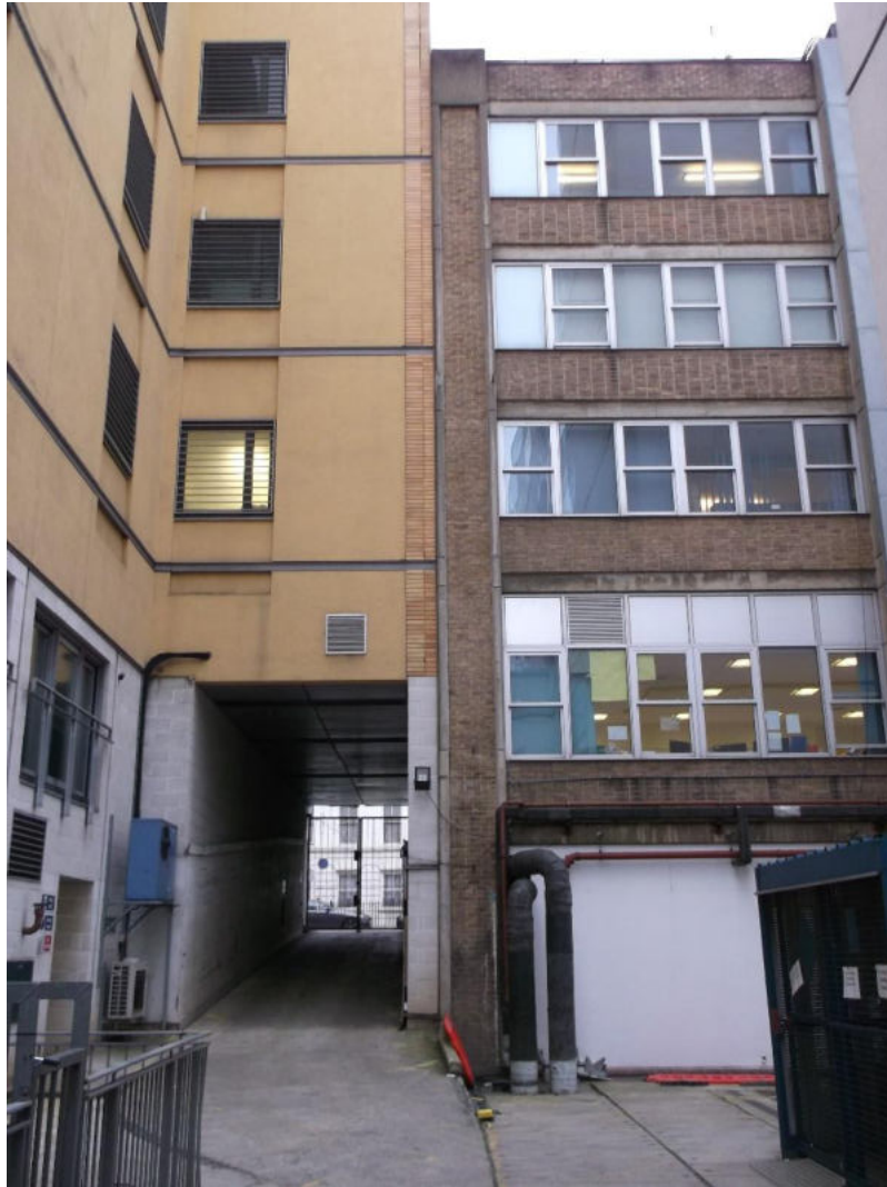
Plate 7: View of the north-east extent of the Front Building from the courtyard and vehicle access to the rear of the building, looking south-east
