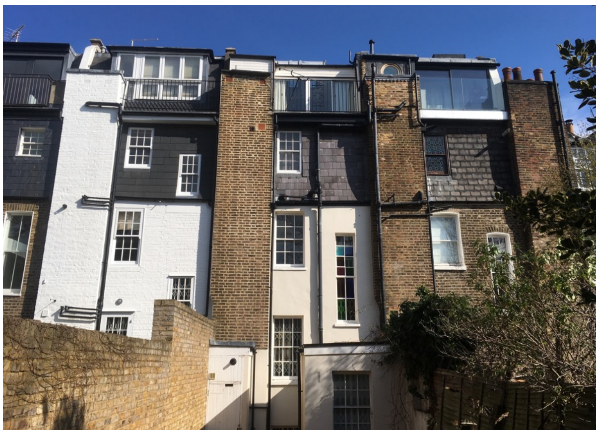
Figure 5: Rear elevation, no. 49 to centre
