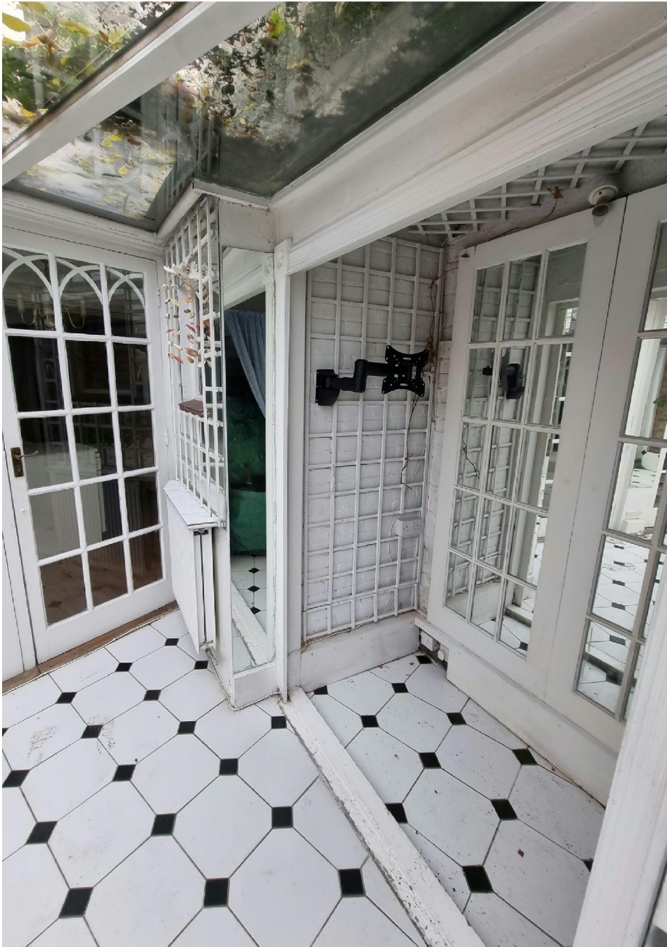
Internal View of Rear Extension
