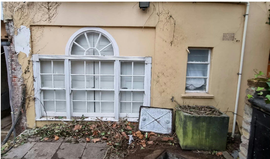
Existing fenestration at lower ground floor - the unusual arched windows sits in an old garage door opening.
