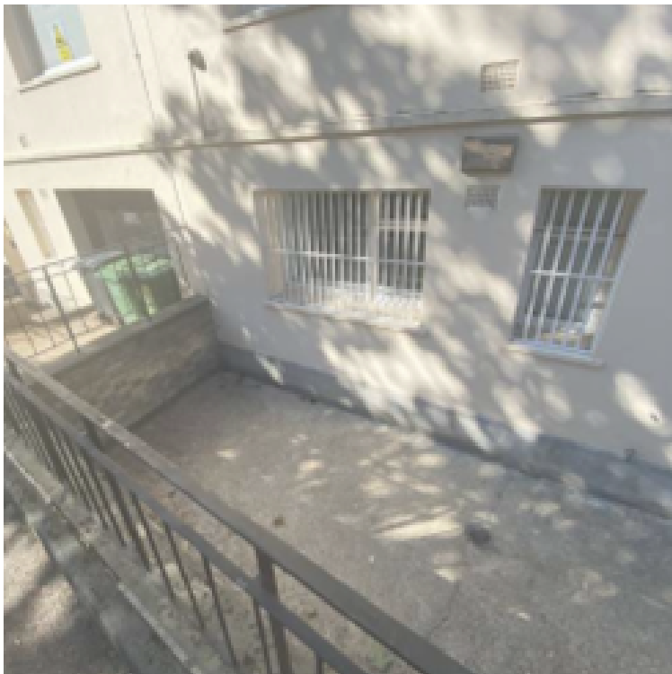
Photo 4: View of existing courtyard at the rear
