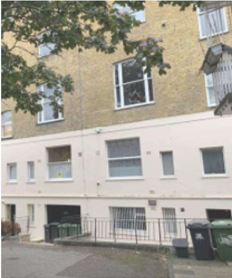
Photo 3: Existing rear elevation from
