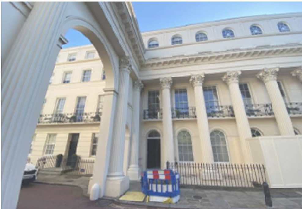
Photo 2: Front elevation of the site from Chester Terrace
