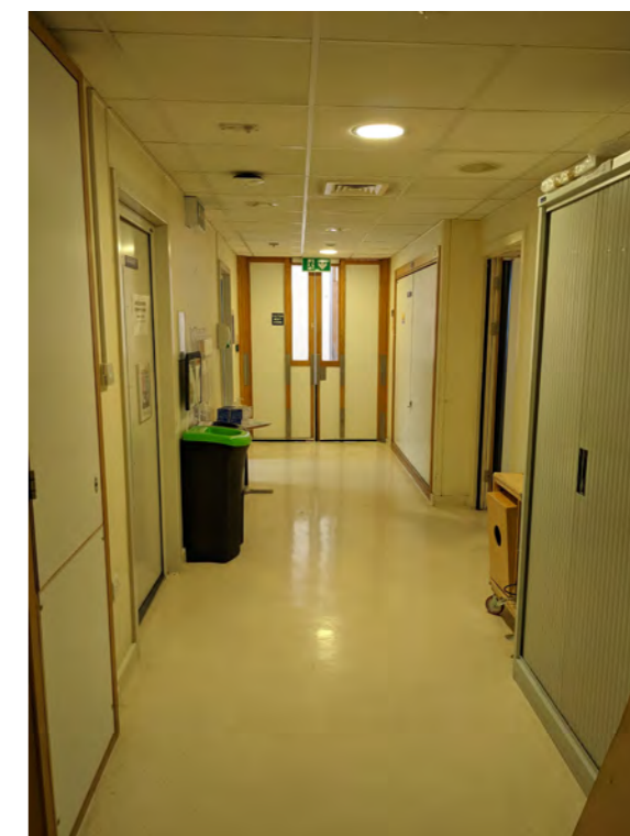
Central corridors without access to daylight
