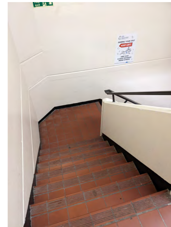
Image of narrow stairs unsuitable for bed movement
