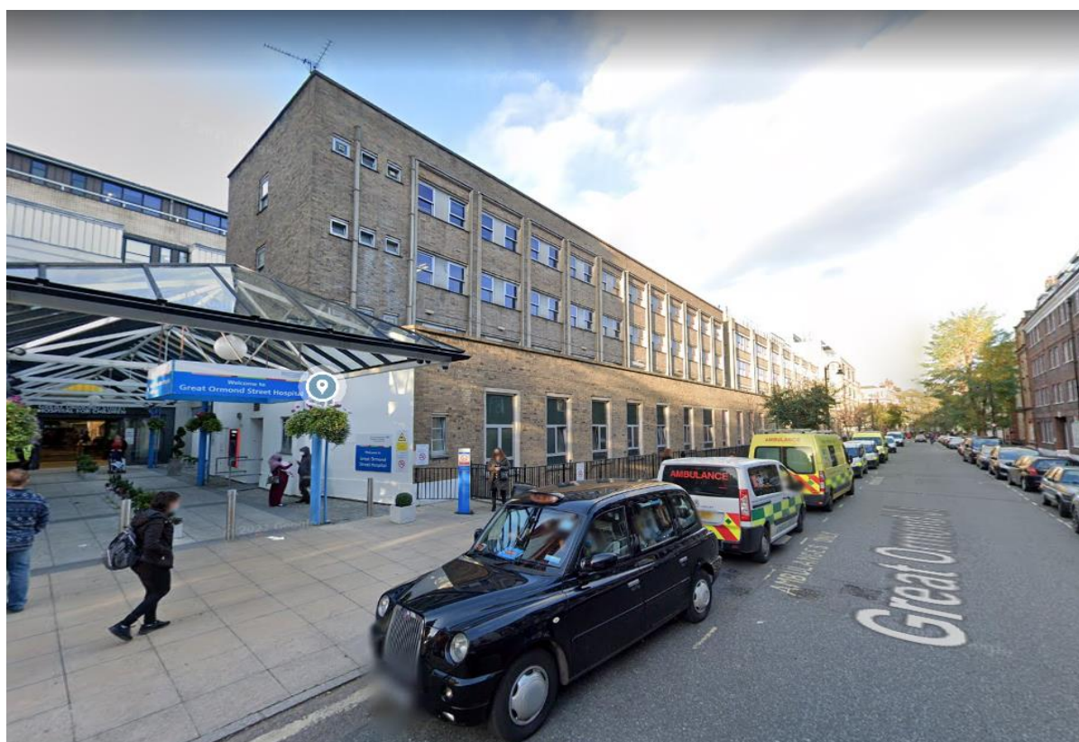
Figure 2.3 View of the current site condition, facing east towards the hospital entrance at Great Ormond Street
