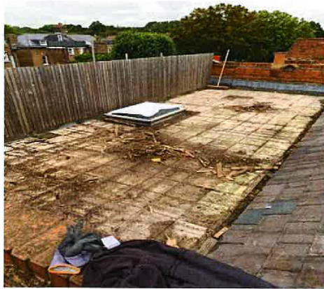
After the strip out of the existing decking we have found asbestos roof tiles
