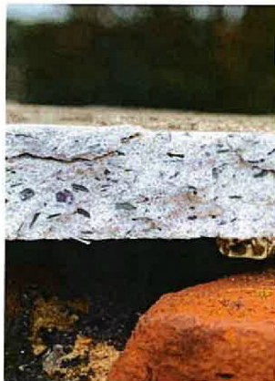
Close up of the asbestos fibres which are compacted in the tiles.
