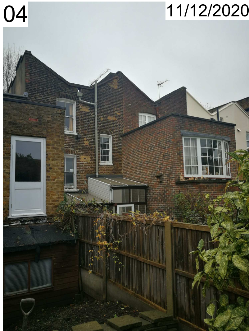
- No.42 (Left Hand Side Neighbour) rear elevation context
