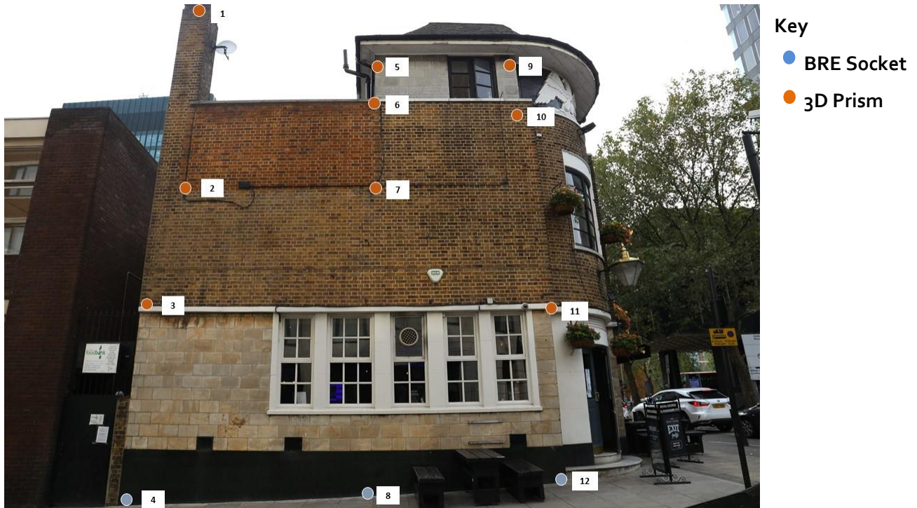
Figure 16. Recommended structural monitoring of north-western façade of Royal George public house.
