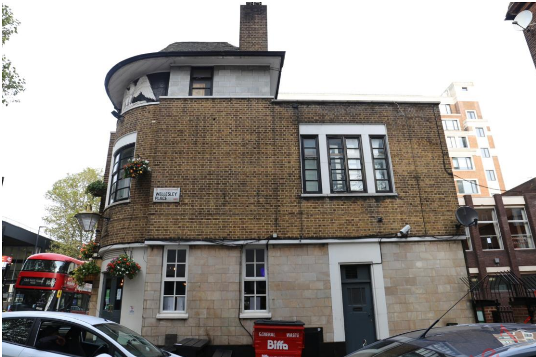
Figure 4. South-eastern elevation. Mott MacDonald (2020).
