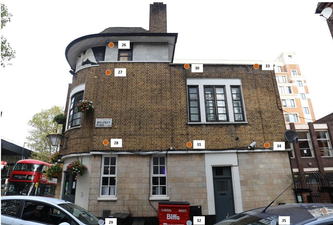
Figure 18. Recommended structural monitoring of south-eastern façade of Royal George public house.
