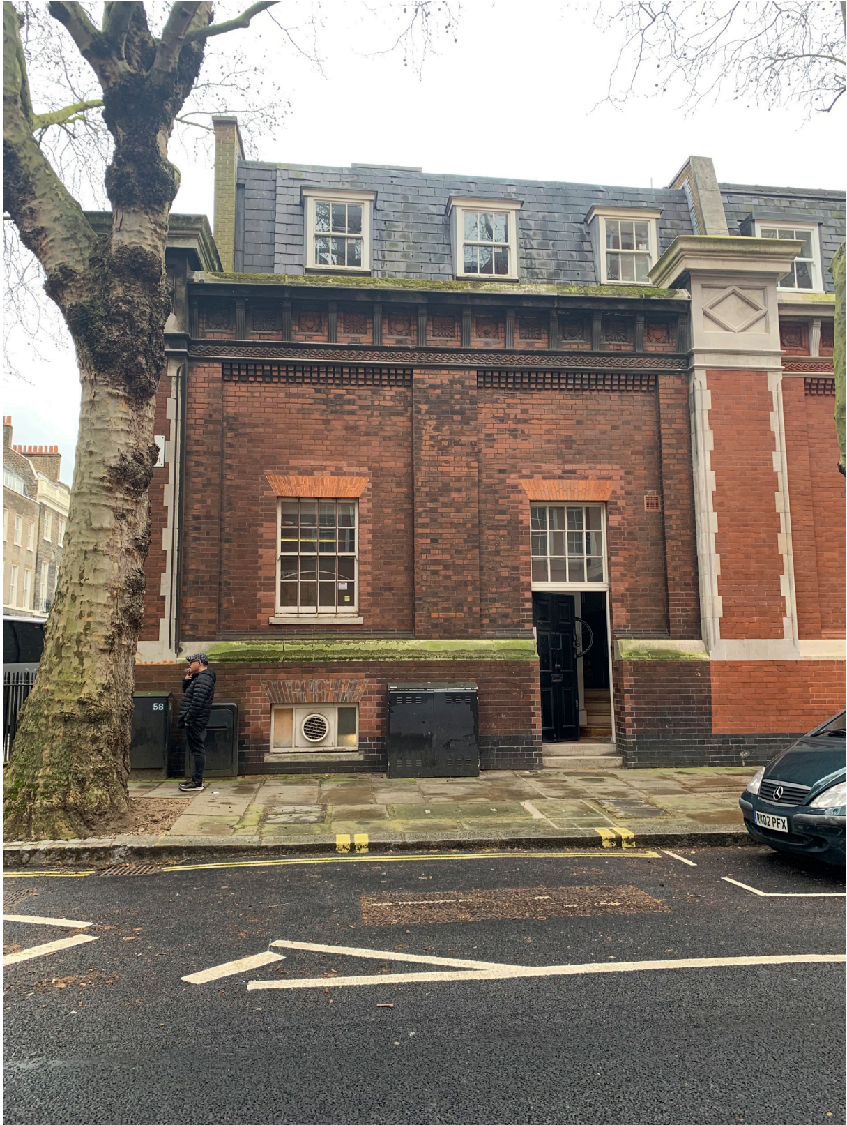
Figure 1: Bedford Avenue Elevation to be cleaned
