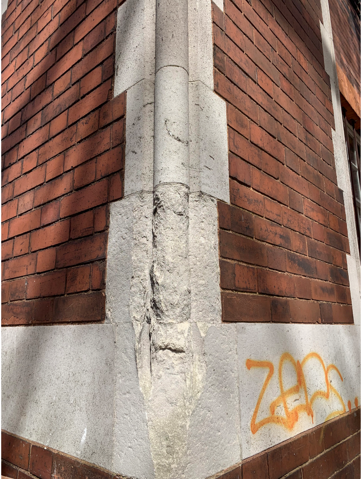
Figure 3: 3.1 - Moulded Stone Indent to corner of Bedford Avenue and Adaline Place. Bottom Course
