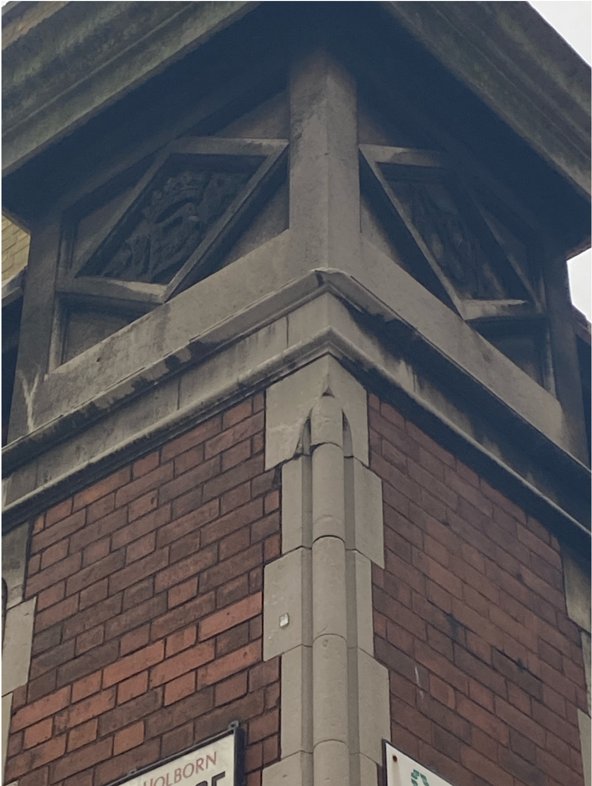
Figure 4: 3.4 - Moulded string course indented to Bedford Avenue
