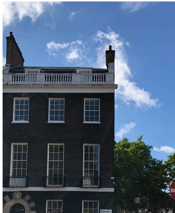
Mews house from Bedford Avenue
