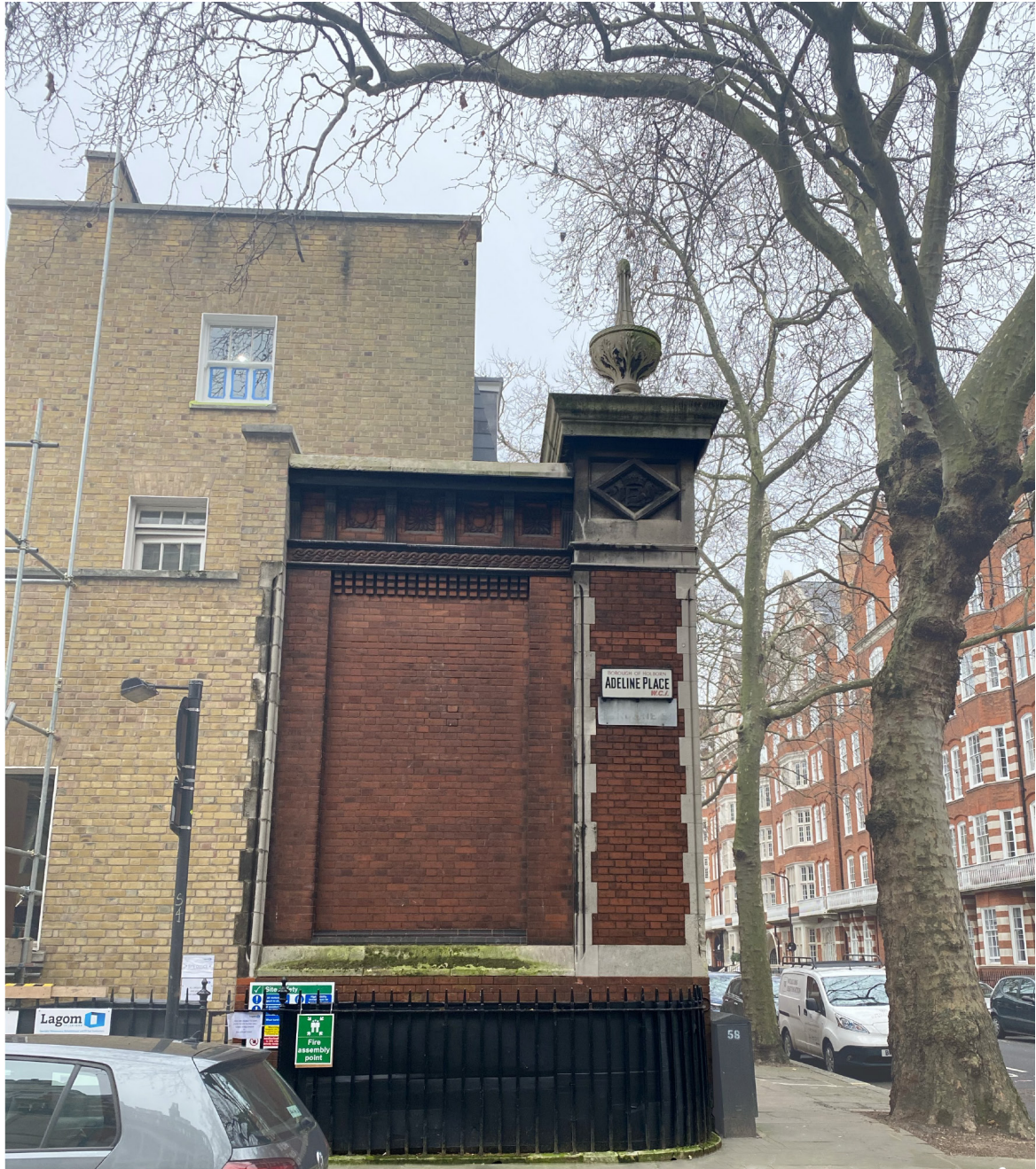
Figure 2: Adeline Place Elevation to be cleaned
