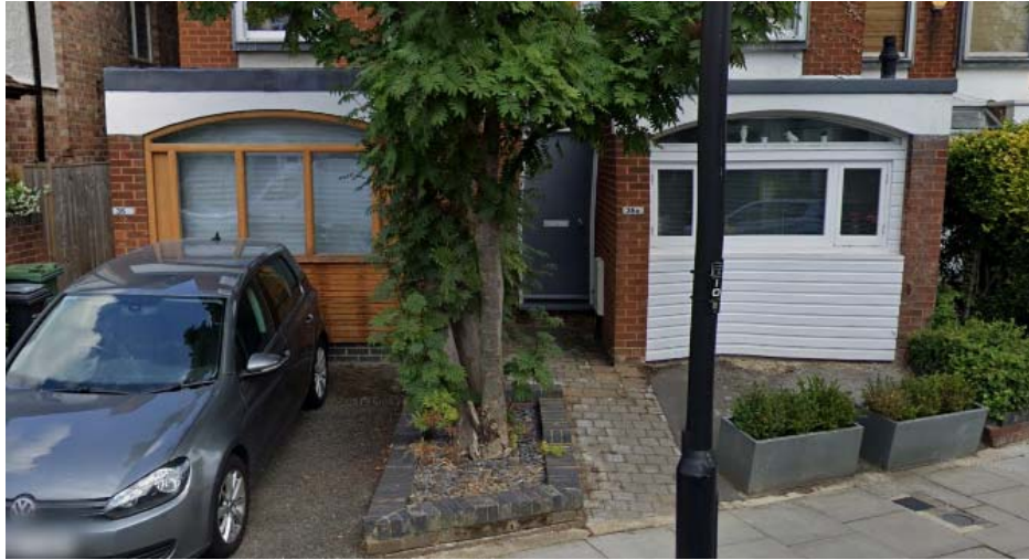
converted garages with arched windows
