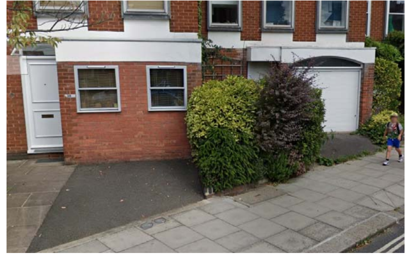
poorly infilled conversion and original arched opening to garage
