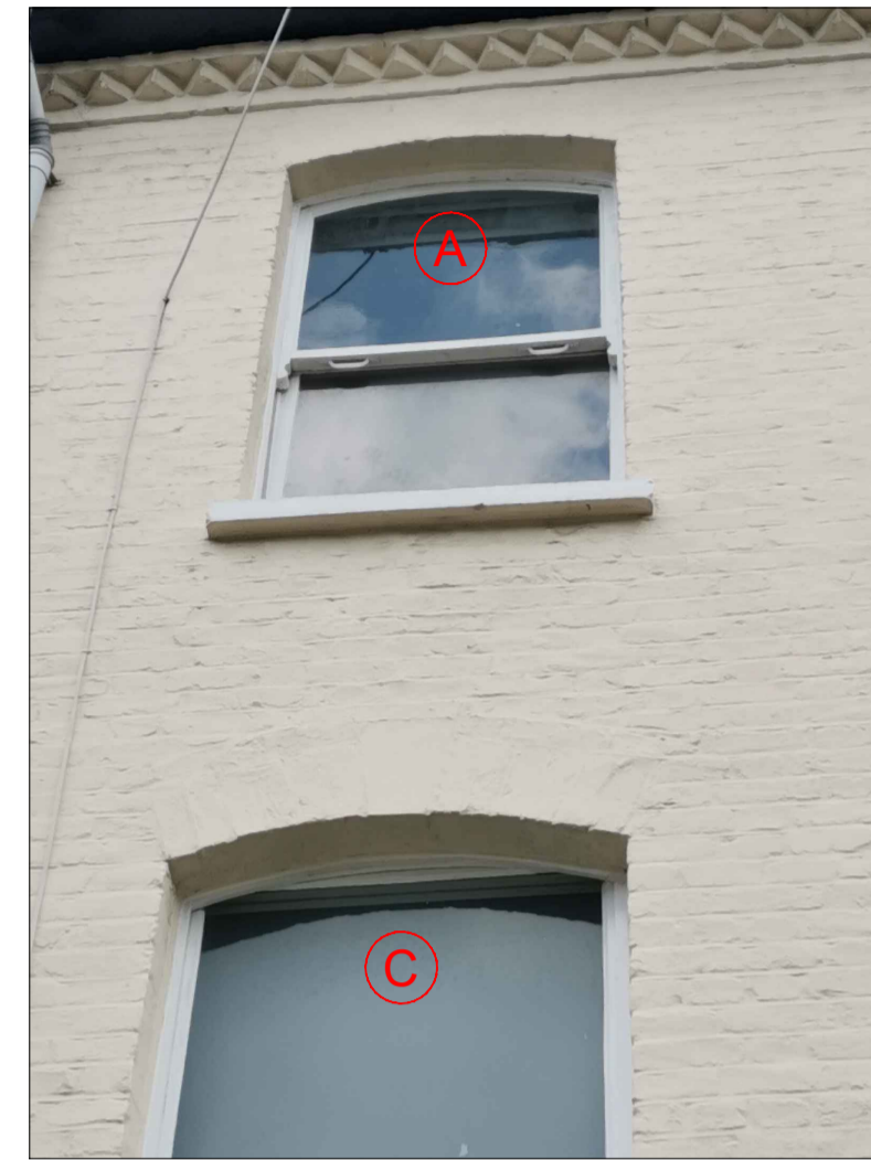
8 EXISTING FRONT ELEVATION 25 LOVERIDGE RD - PHOTO NOT TO SCALE
