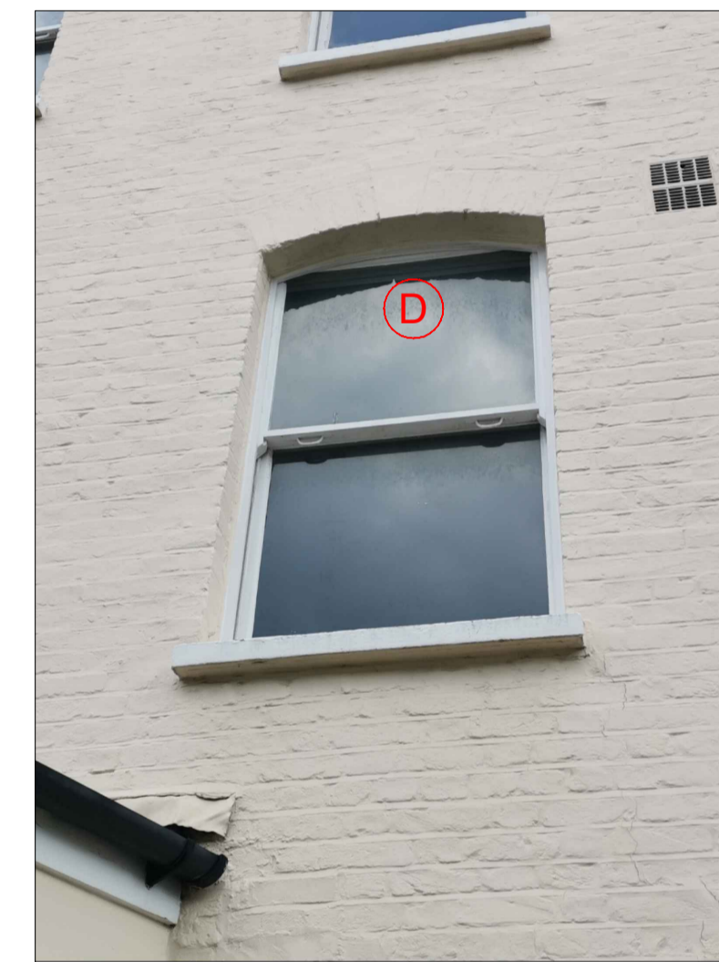
11 EXISTING FRONT ELEVATION 25 LOVERIDGE RD - PHOTO NOT TO SCALE
