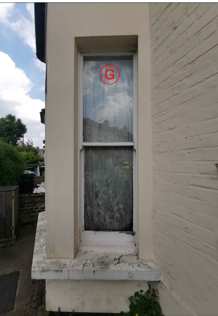
15 EXISTING FRONT ELEVATION 25 LOVERIDGE RD - PHOTO NOT TO SCALE
