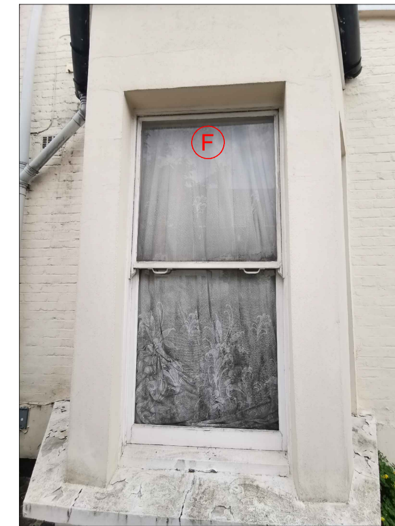
14 EXISTING FRONT ELEVATION 25 LOVERIDGE RD - PHOTO NOT TO SCALE
