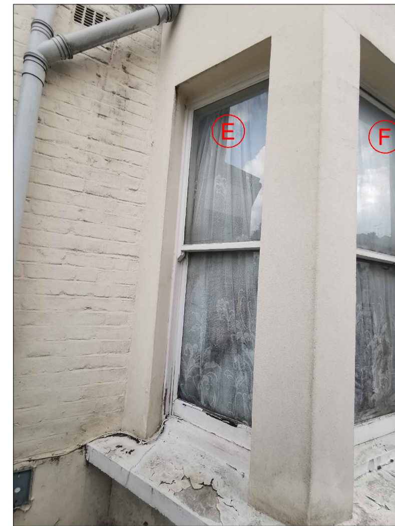
13 EXISTING FRONT ELEVATION 25 LOVERIDGE RD - PHOTO NOT TO SCALE
