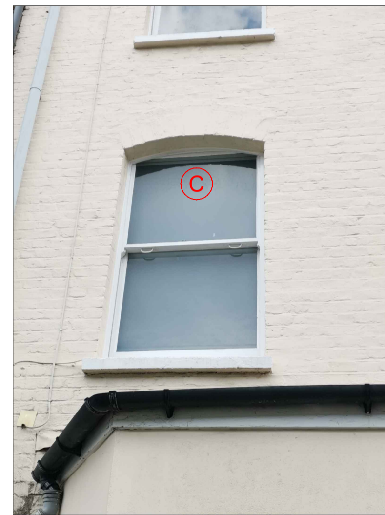
10 EXISTING FRONT ELEVATION 25 LOVERIDGE RD - PHOTO NOT TO SCALE
