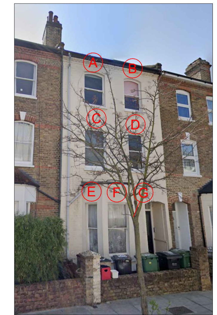
12 EXISTING FRONT ELEVATION 25 LOVERIDGE RD - PHOTO NOT TO SCALE
