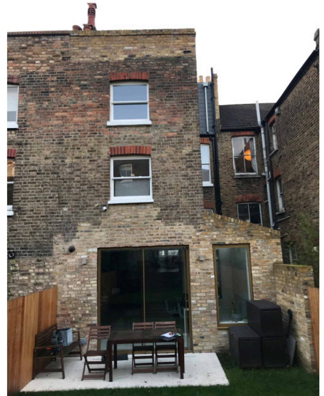
Rear elevation of 13 Kylemore Road
