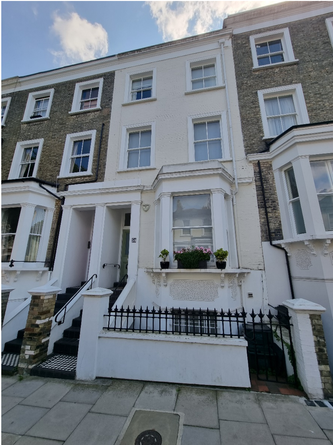
Figure 2 - Photograph of the existing front facade
