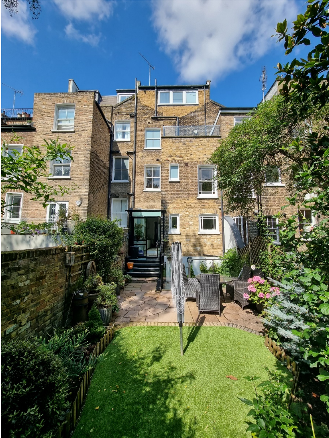
Figure 4 - Photograph of the existing rear facade of No.50
