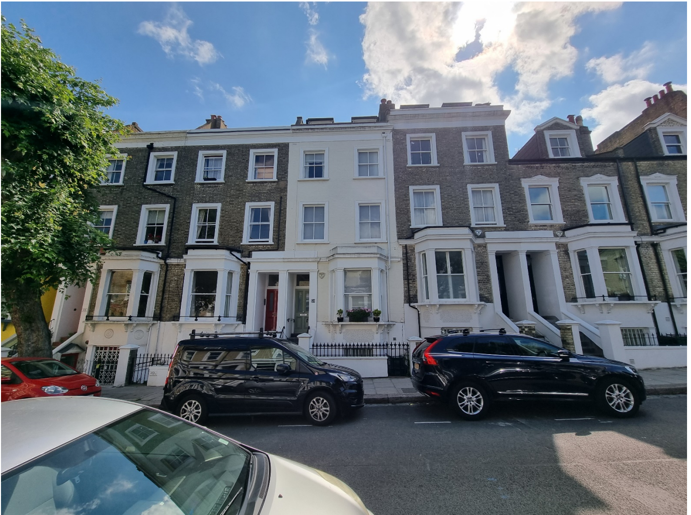
Figure 3 - Photograph of the existing house at No.50 from across the street showing its relationship to the terrace row
