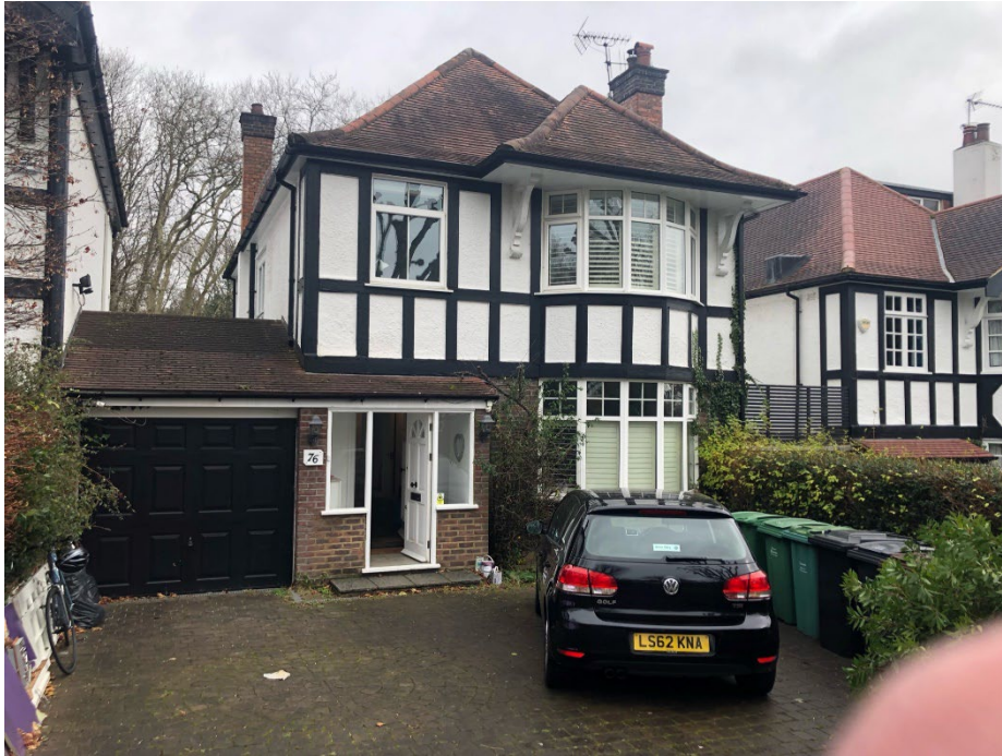
Photos of Existing Building- Front
