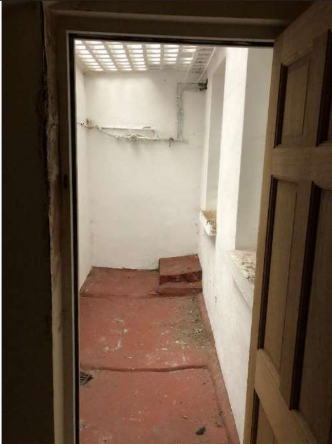
Basement Passage under pavement lights, looking North
