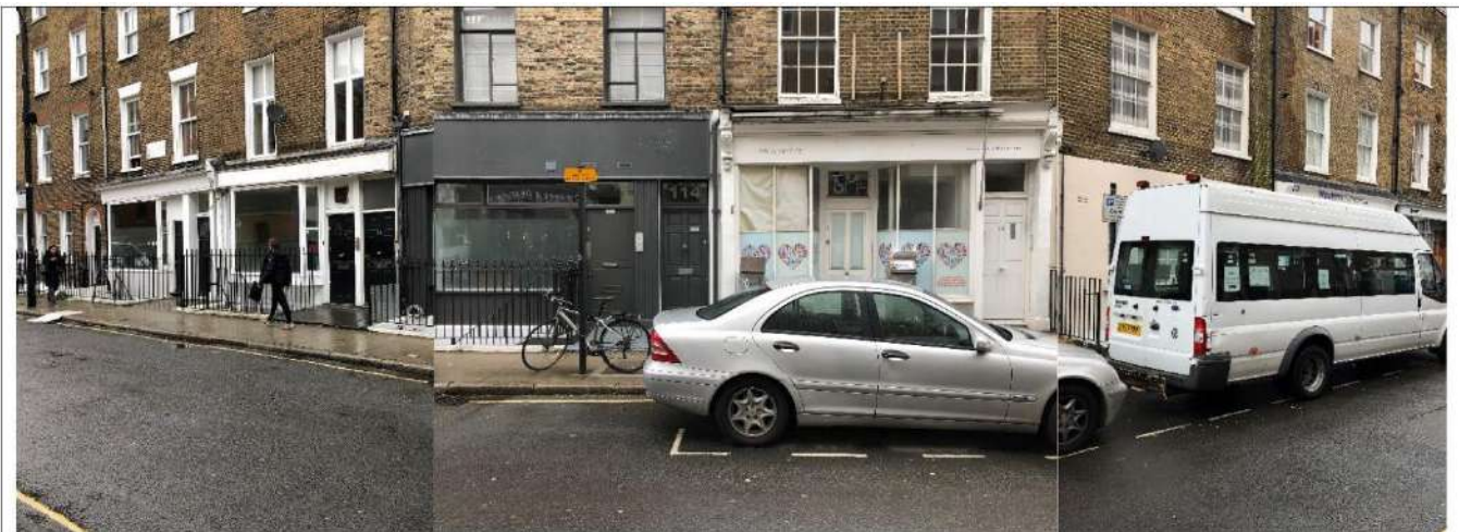
View from Cleveland Street
